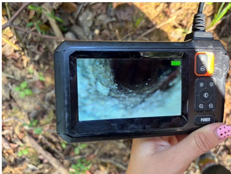
View of chimney with endoscope
